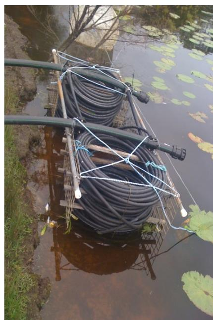
Figure 4 Heat exchange loops prior to placement in dam
