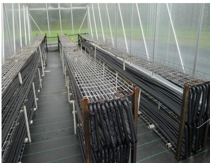
Figure 3 Hydronic heating system in demonstration greenhouse
