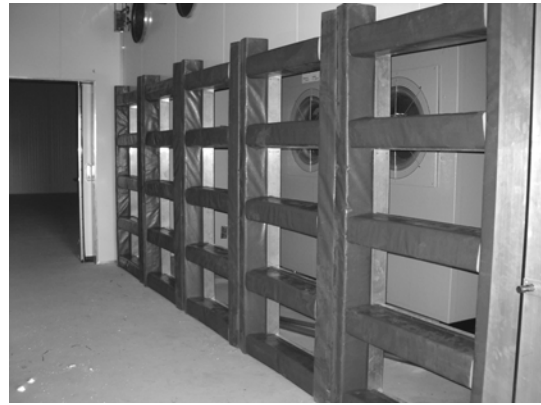
Figure 5b. Internal view of empty chamber
